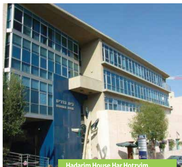
Hadarim House Har Hotzvim, Managed and Maintained by Natam
